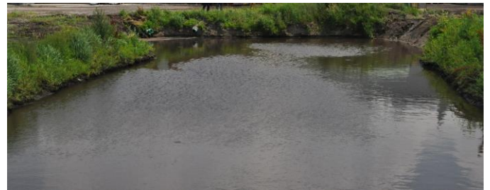
Figure 1: An example of a clay-lined settling pond
