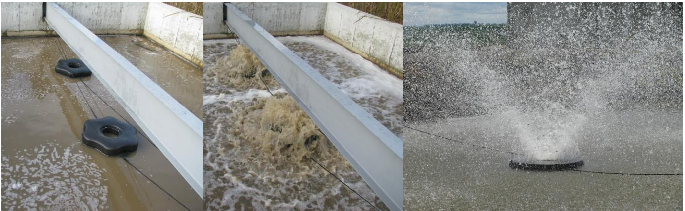
Figure 3 (from left to right) installed surface aerator, surface disturbance, and fountain-style aerator
