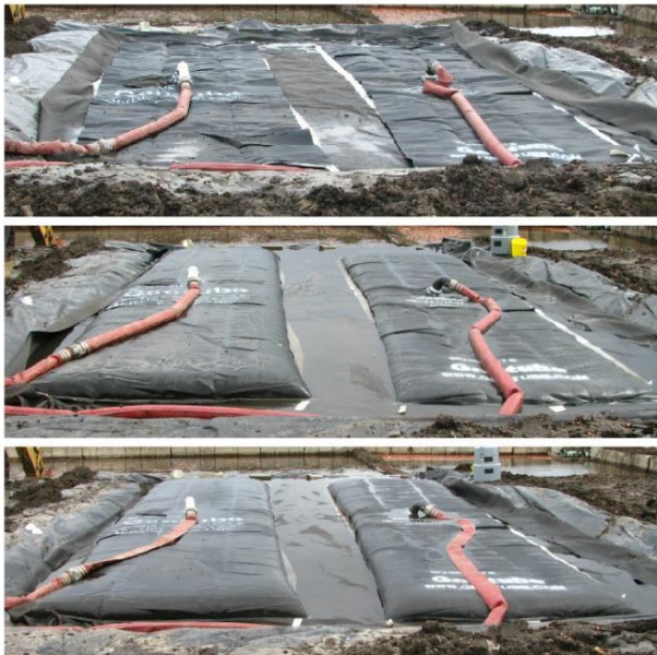
Figure 2: Time lapse photos of the Geotubes® at the beginning (top), mid-way (middle), and end (bottom).
