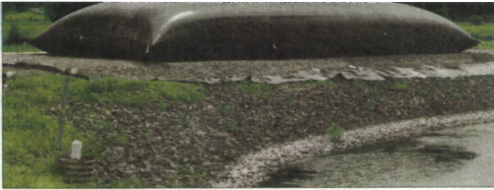
Geotube dewatering system
